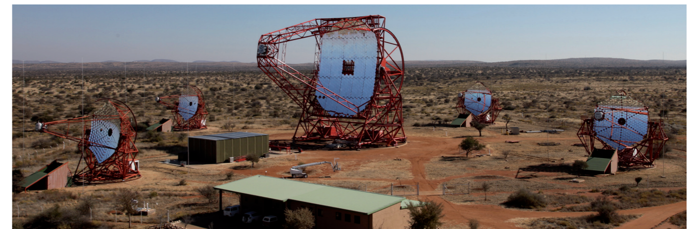
Fig. 2: The new 600 \text{ m}^2 H.E.S.S. II telescope at the center of the H.E.S.S. telescope array.
