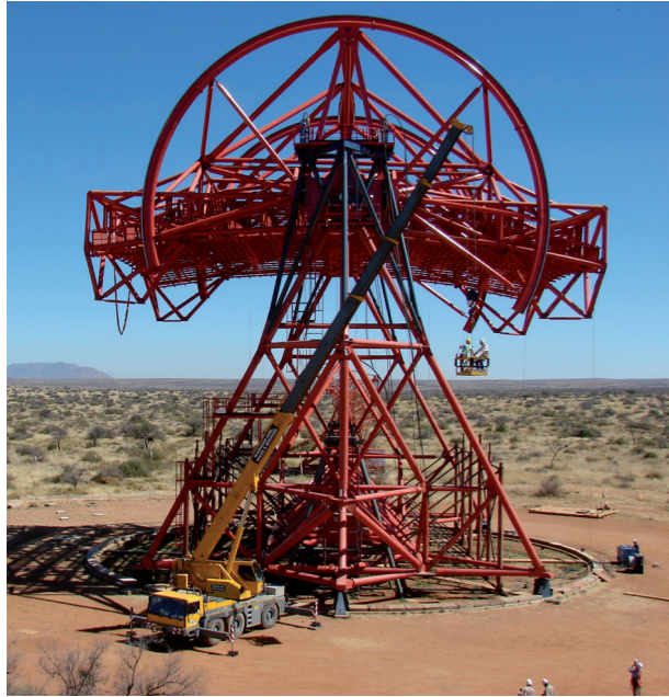
Fig. 3: The “Big Lift”: One of the most critical moments in assembling the telescope was the lifting of the dish.
